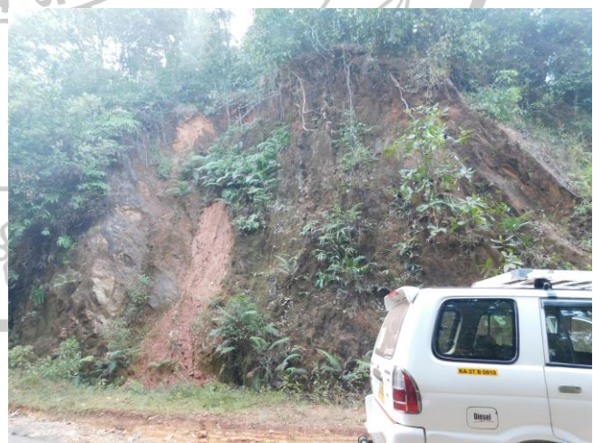
Photo 12: Landslide along the road section near Herur.
